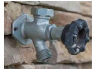
Here is a picture of an atmospheric vacuum breaker (AVB) installed on the bib.
